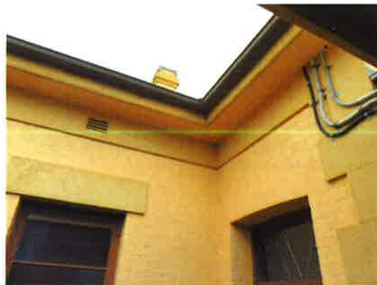
Figure 3.10 Detail of original lockup building showing rendered detail, eaves and chimney.
