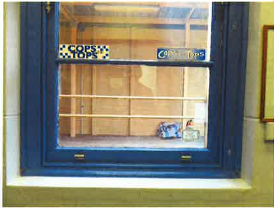
Figure 3.23 Windows with horizontal glazing bars appear to have been inserted into original openings during the 1940s.
