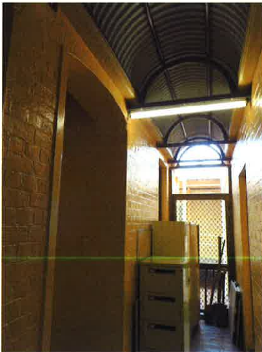
Figure 3.13 Breezeway between original building (left) and 1990s addition (right). The original entrance to the former lockup keeper's residence is on the left. The breezeway replaces the earlier verandah.
