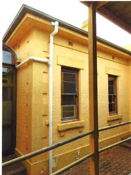
Figure 3.8 Original entrance front (east elevation) to lockup and lockup keeper's residence, showing rendered detail on front façade, including quoins, plinth, top band, sills and lintels.
