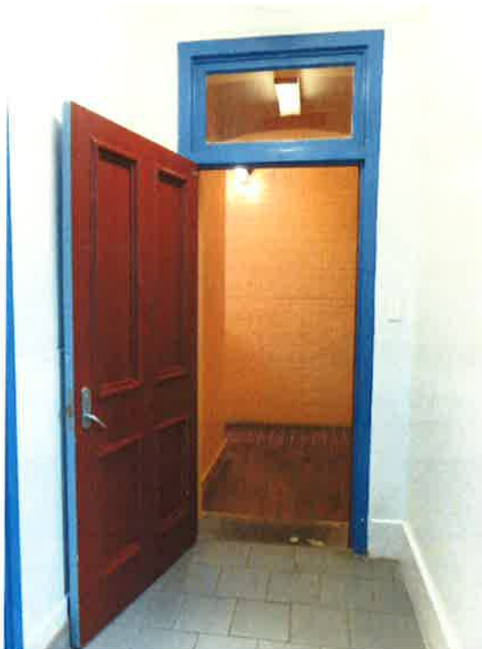
Figure 3.15 Original entrance door to former lockup keeper's residence looking out to breezeway from entrance hall. The original timber floor has been replaced with a concrete slab, the skirting is rendered and the ceiling is plasterboard.
