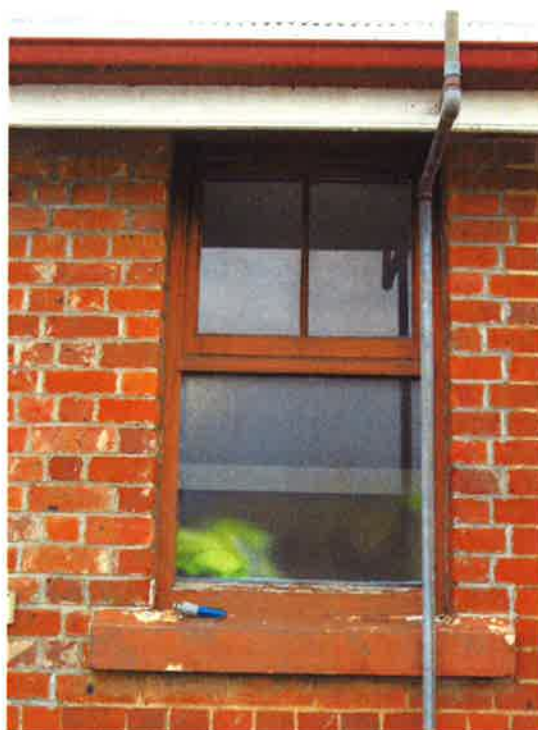
Figure 3.38 Original window opening to former stables (south elevation). Glass louvres have been replaced with a fixed sash.
