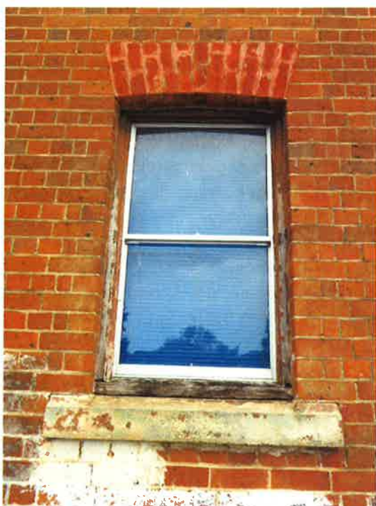
Figure 3.37 Original window opening in the western elevation, showing tuckpointed head and rendered sill. The window has been replaced in aluminium.
