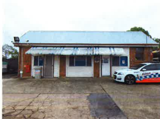
Figure 3.36 The large openings from when the stables were converted to garages during the 1940s have been infilled to enable the building's use as offices.
