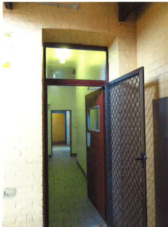
Figure 3.16 Rear door to the former lockup. The opening is original, but the door has been altered. The original floor has been replaced with concrete and tiled.
