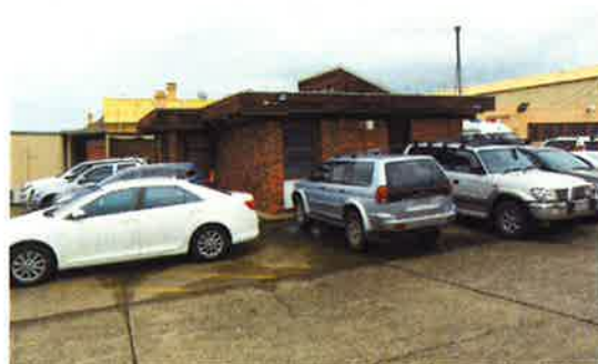
Figure 3.30 The 1968 addition is of brick construction with a flat roof, featuring deep weatherboard fascias and concealed gutter detail.
