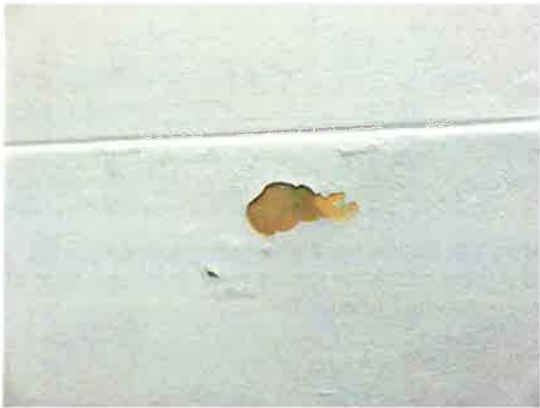
Figure 3.25 Evidence of early colour schemes survive below the existing paint finishes.
