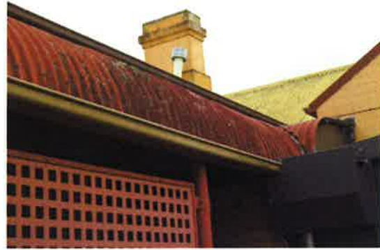
Figure 3.12 Bullnose verandah roof bellows to 1990s additions. The chimney is original.
